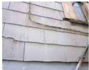
Asbestos cladding.
