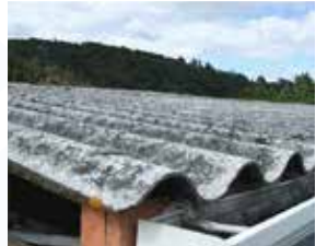
Asbestos roofing.
