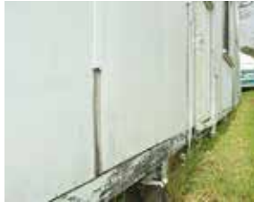
Asbestos joints.
