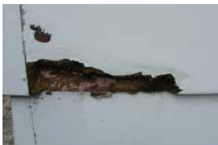
Photos of Oil Tempered Hardboard ('Weatherside')
