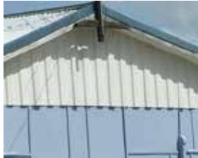
Asbestos cladding.
