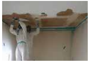
Asbestos ceiling removal.
