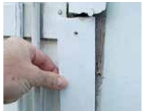
Asbestos joiner.
